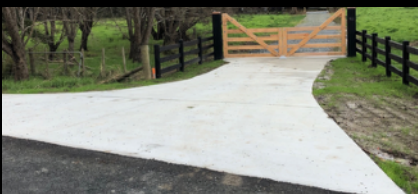
Auckland Transport Compliant Vehicular Crossing
